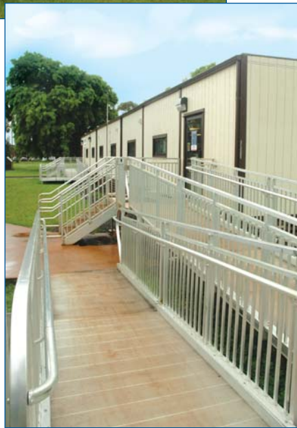
Below - Ramp with stair system footprint. Additional stairs can be added to the system.
